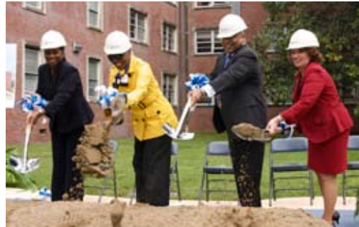
Tennessee State University's president, administrators and faculty break ground on a new $1 million addition to the university's dental hygiene clinic
